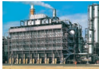
68,750 Nm³/Hr H₂ Plant
