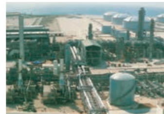
2,500 T/D Methanol Plant
