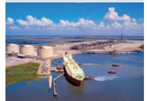
Courtesy of Cameron LNG, LLC
