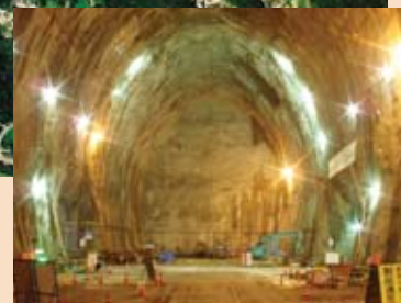
LPG岩盤貯槽
