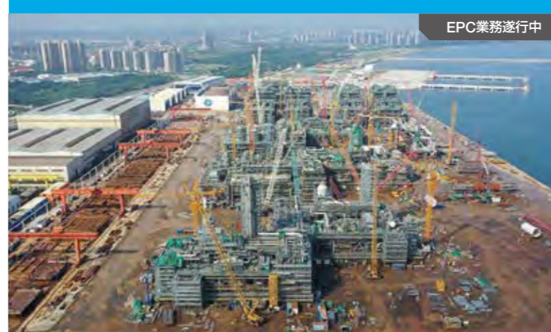
Overview of ongoing Module Fabrication
