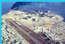
1976 Completion of LNG plant for Abu Dhabi Gas Liquefaction in UAE
