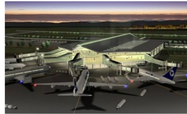
▲ Construction of New Ulaanbaatar International Airport in Mongolia
