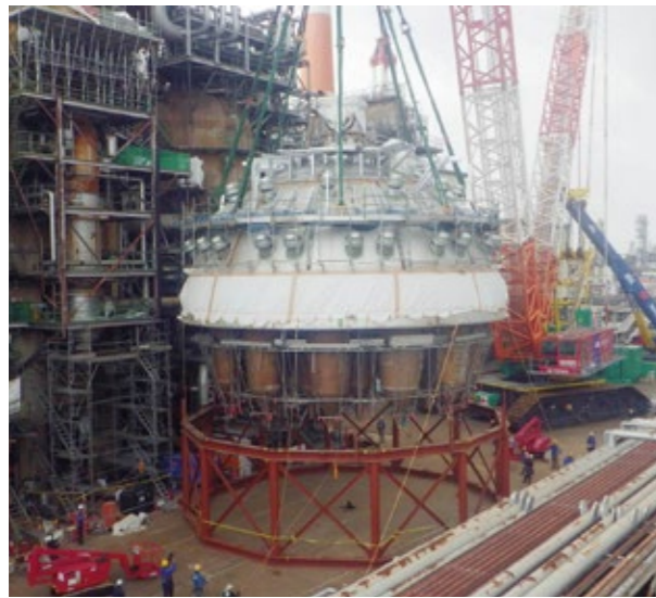
▲ RFCC Unit Regenerator cyclone system unit renewal work
