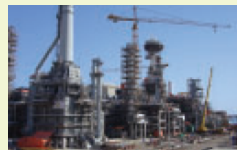
Work proceeds at an LNG plant in Oman.
