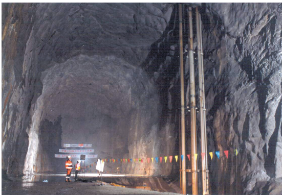
The LPG storage facility and the ingress shaft
