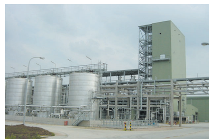
Converted epoxy resin plant for Dow Chemical (Zhangjiagang, China)
