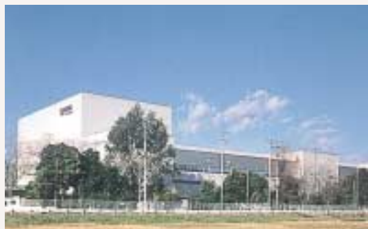
Chiyoda completed a new solid dosage drug production facility – the largest such facility in Japan – for Nippon Shinyaku.
