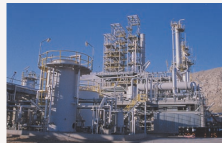
A view of CCR reforming units constructed in a Turkmenbashi refinery
