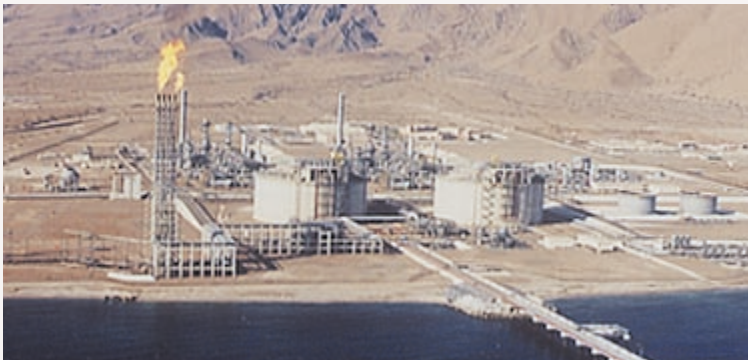
Bird's-eye view of the Oman LNG complex, Qalhat, Oman
